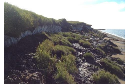
Thawing permafrost leading to rapid erosion in northern Canada
