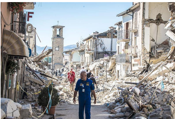
Damage in the town of Amatrice following the August 2016 Central Italy Earthquake
