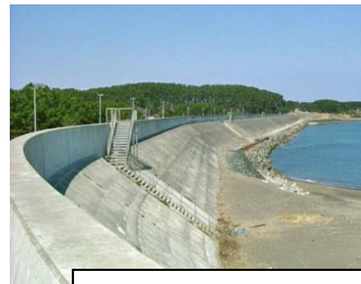
Tsunami walls and closable sluice gates can offer protection for some, but not all parts of the coast
