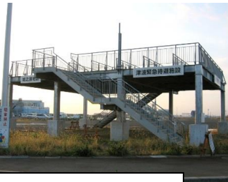
Tsunami shelters provide limited protection from smaller waves for those who can't evacuate
